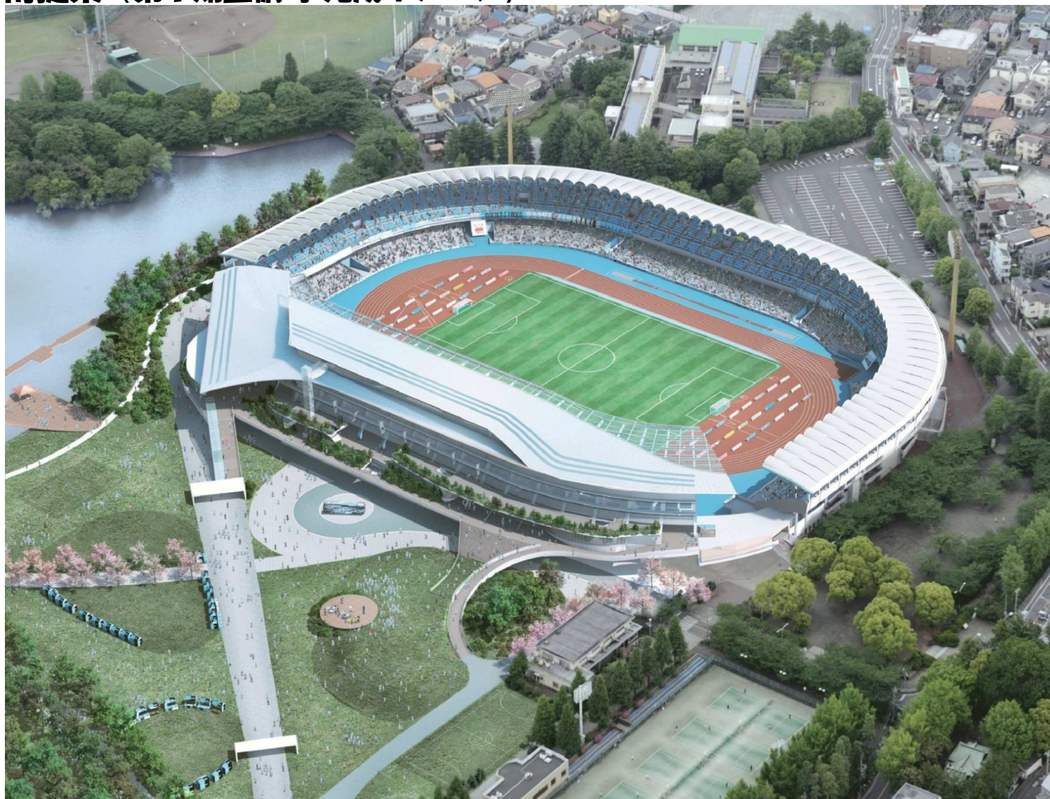
Reconstruction Work of Todoroki Stadium Grandstand
