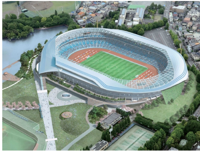
Reconstruction Work of Todoroki Stadium Grandstand
